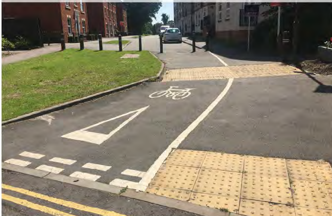
Figure: Example of off-road cycle track along line of a footpath, that crosses the footway to join the road. This type of route can also cross minor roads with priority for the cycle track, using a flat top road hump. (Photograph by Adrian Lord)
