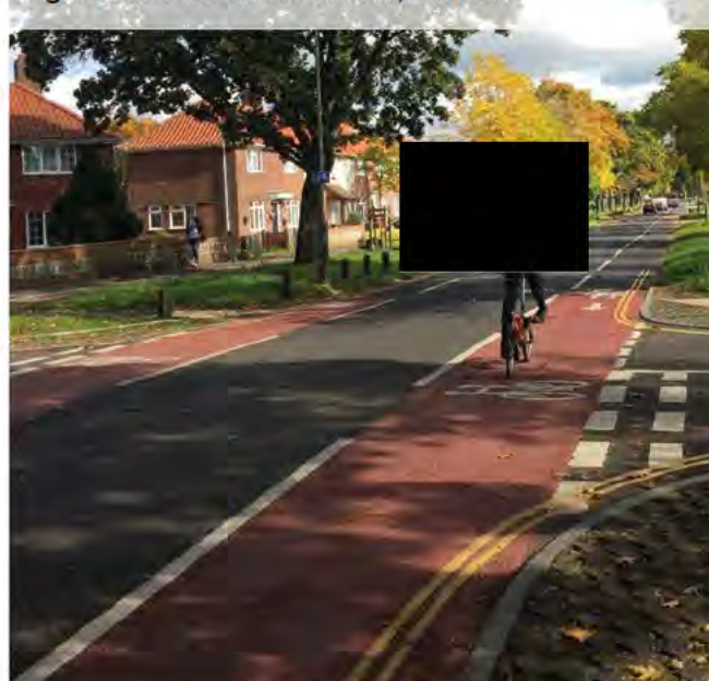
Figure 6.21: Centre line removal, Norwich
