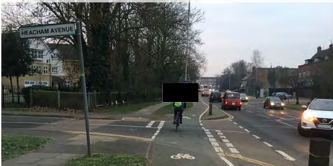
Figure 10.16: Partial set back, marked priority crossing, Hillingdon
