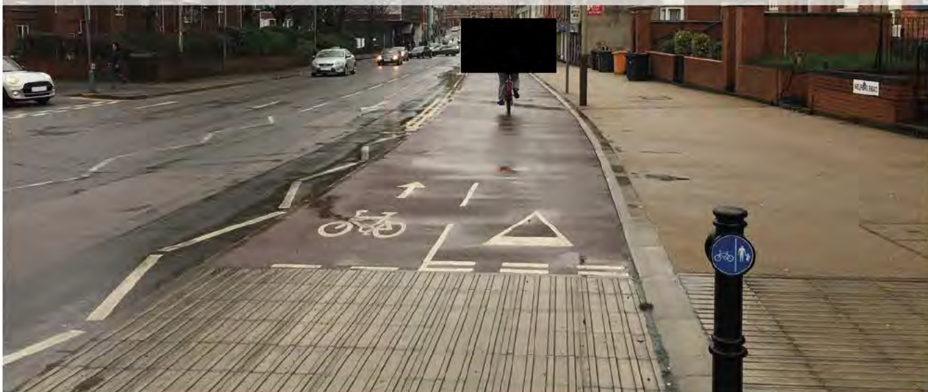
Figure 9.8: Correct use of tactile paving and low kerbs at start of segregated area, Leicester
