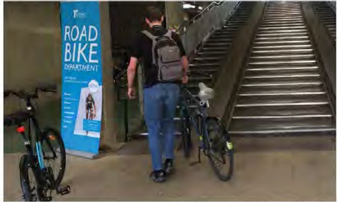
Figure 11.5: Public cycle hub at Cambridge station. Note the wheeling ramp to access cycle parking upstairs: such ramps may not be suitable for “non-standard” cycles, but here dedicated parking provision for these is available at ground level, and generally well-respected
