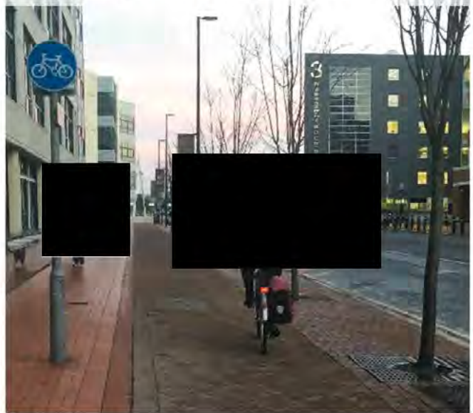
Figure 6.14: Cycle track with sign to TSRGD diagram 955
