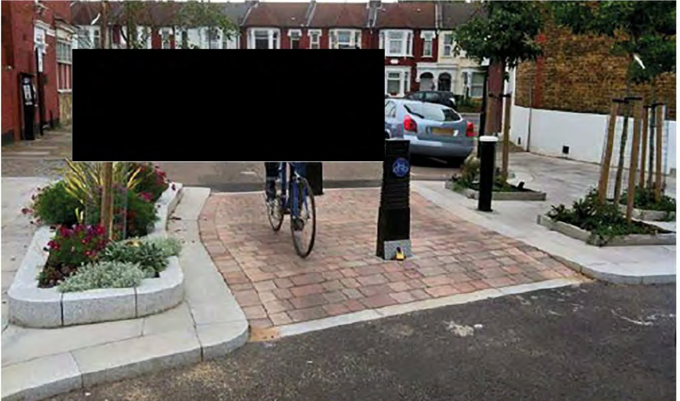
Figure 7.1: Simple modal filters can reduce through traffic while retaining cycle and pedestrian access. The central position enables kerbside car parking to be provided without blocking the facility, and the lockable bollard enables emergency access, Haringey.
