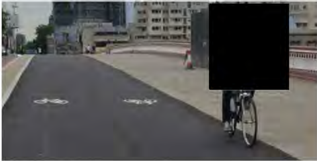
Figure 6.6: Footway-level cycle track with different surface materials to footway, London
