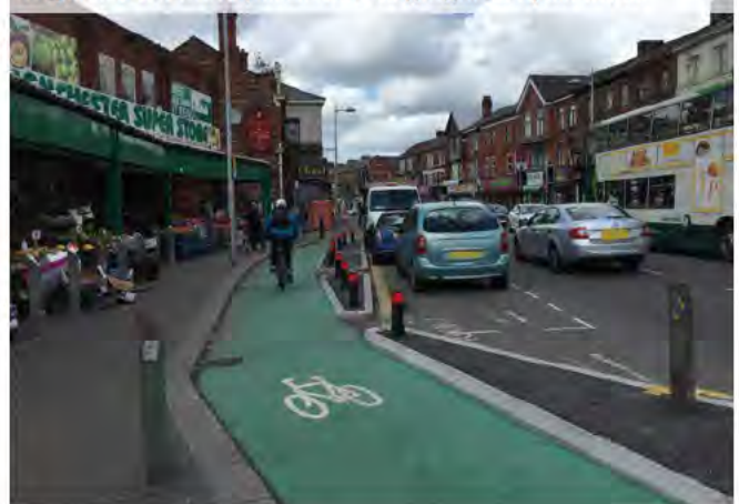
Figure 1.10: Example of kerb-segregated cycle track
