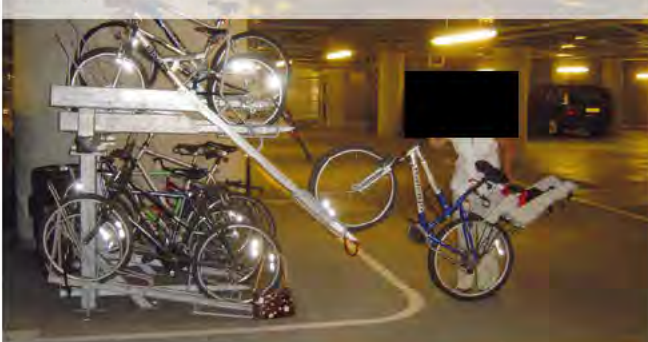
Figure 11.14: Basement cycle parking in residential development, London
