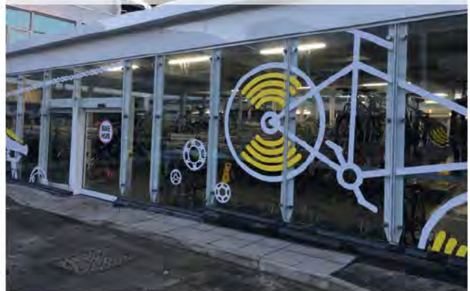
Figure 11.6: Secure cycle-hub (pass holders only) at Coventry station
