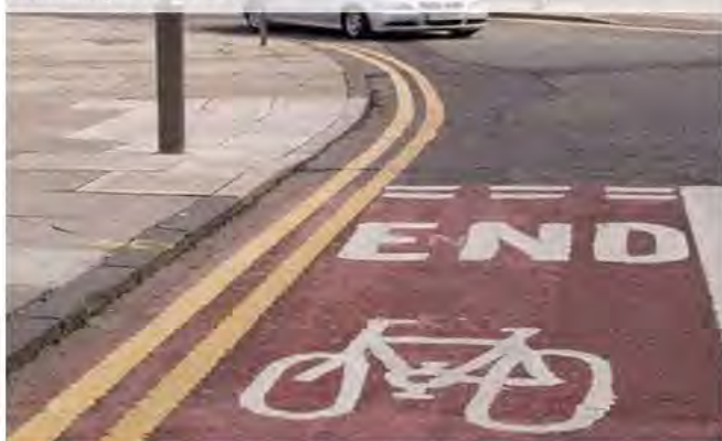
Figure 6.26: The END marking (TSRGD diagram 1058) and give way marking (TSRGD diagram 1003B) should not normally be used.
