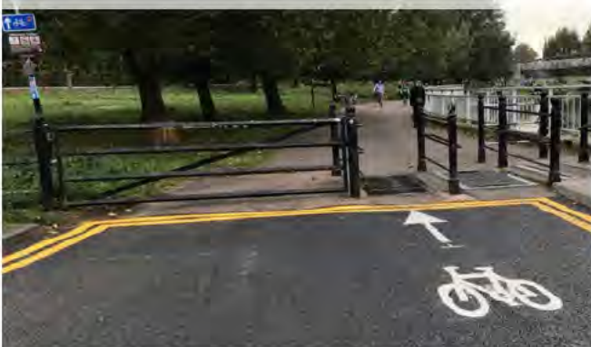
Figure 8.4: Cattle grid access control, Cambridge
