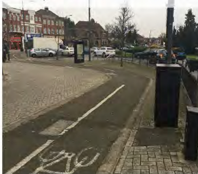
Figure 10.36: Footway-level cycle track around large roundabout, Harrow
