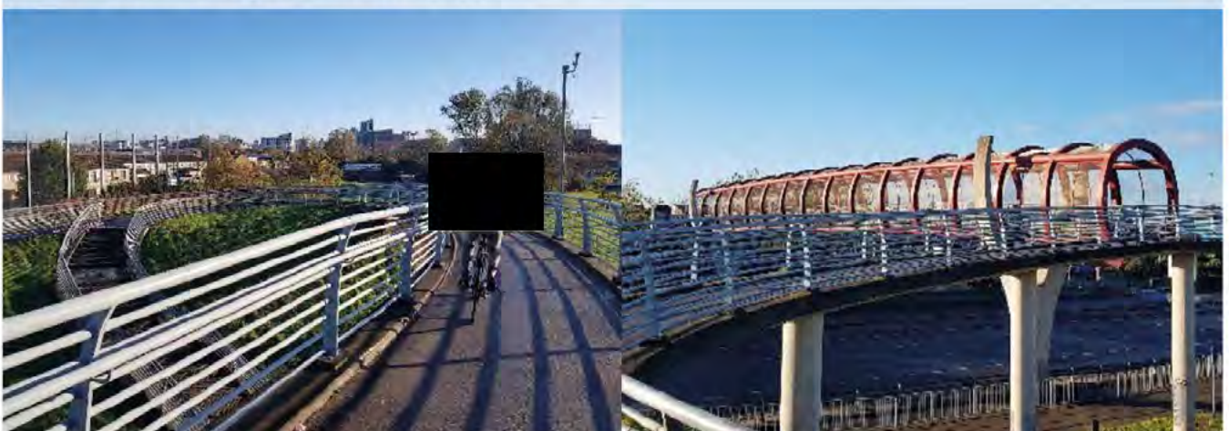
Figure: 10.53: Overbridge with curved ramp approach, Belfast
