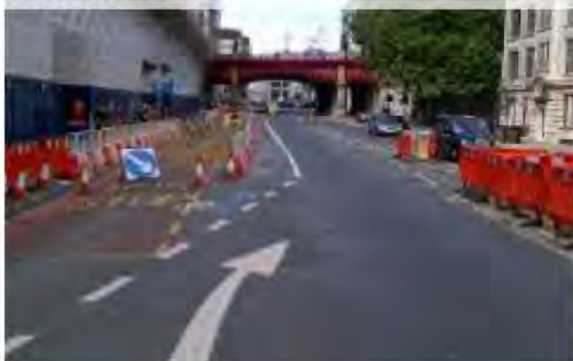
Figure 13.7: Warning signs and temporary markings at construction site
