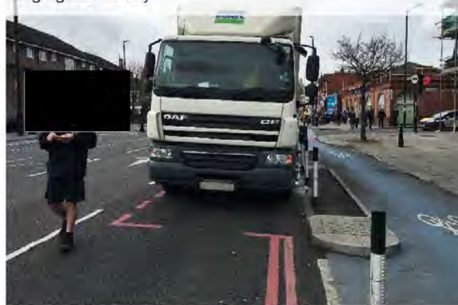
Figure 6.18: Local kerbed island for servicing across light segregation facility
